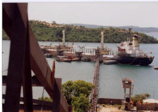
PIPE CONVEYOR INSTALLATION - TRINCOMALEE
