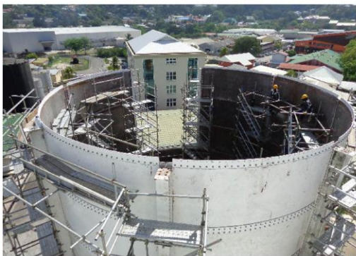
4000T SILO ERECTION AT LAFARGE CEMENT COMPANY SEYCHELLES
