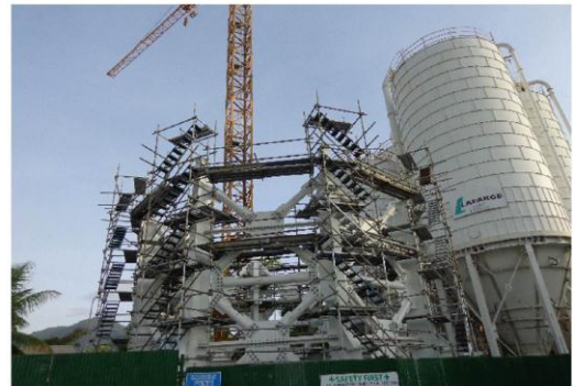
4000T SILO ERECTION AT LAFARGE CEMENTS MAYOTTE S.A. - MAYOTTE
