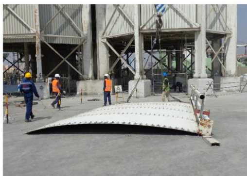
DISMANTLING OF STEEL SILOS IN PORT SUDAN
