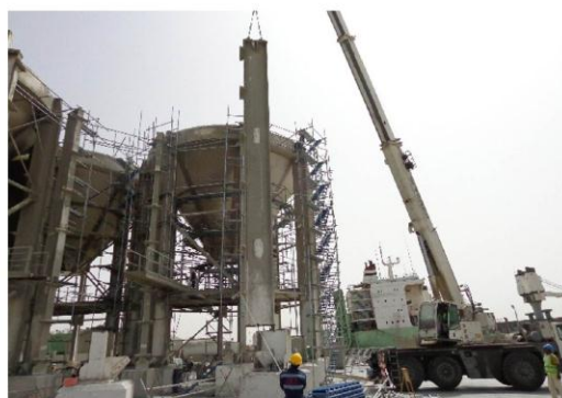
DISMANTLING OF STEEL SILOS IN PORT SUDAN
