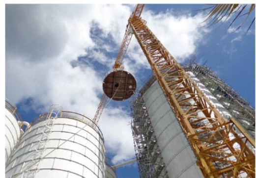
4000T SILO ERECTION AT LAFARGE CEMENT COMPANY SEYCHELLES
