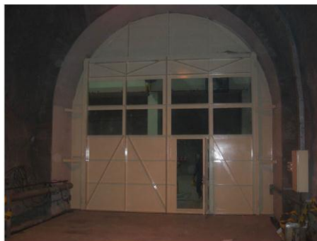
UPPER-KOTMALE HYDRO POWER PLANT - TUNNEL GATES
