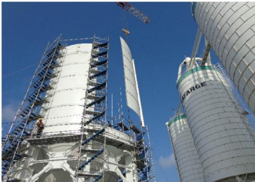
4000T SILO ERECTION AT LAFARGE MALDIVES CEMENT - MALE
