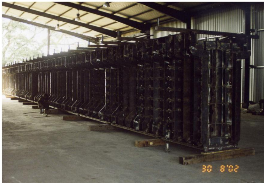
STEEL FORM FOR MAIN GIRDER - GAMPOLA BRIDGE
