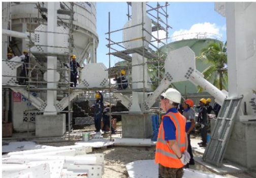
4000T SILO ERECTION AT LAFARGE CEMENTS MAYOTTE S.A. - MAYOTTE
